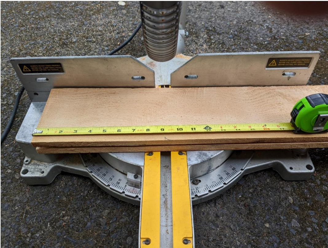
Figure 2 - Cut the top pieces
